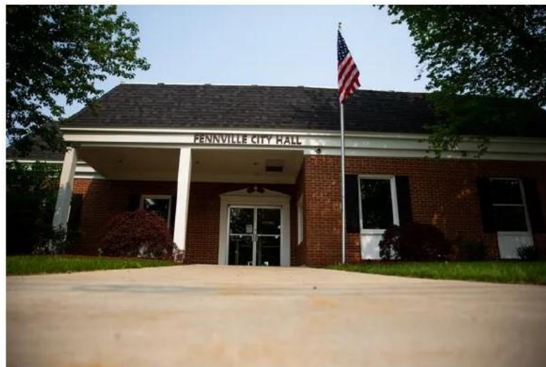
Fennville City Hall is pictured May 17, 2023. Four seats on the city commission will be write-in only this November. Cody Scanlan/Holland Sentinel
