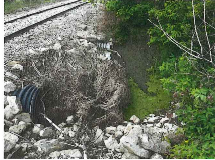
Upstream side of Railroad Tracks
