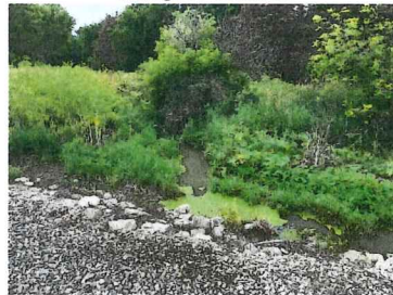
Looking upstream (towards 47th St) where Hamilton Drain first approaches railroad tracks
