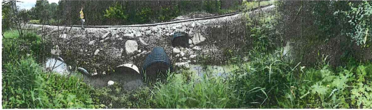
5 culverts underneath track (view from downstream side)
