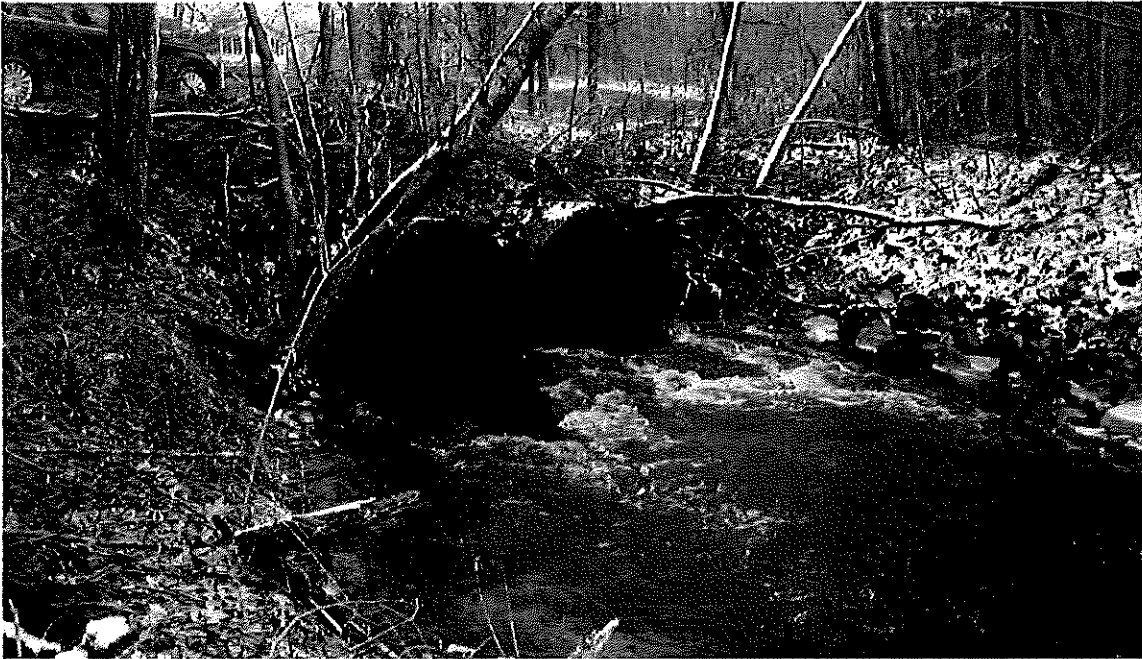
Picture No. 1 shows the southern end of the three steel culverts under Garbow Road. Dead trees have fallen across this outlet end of the eastern culvert.
