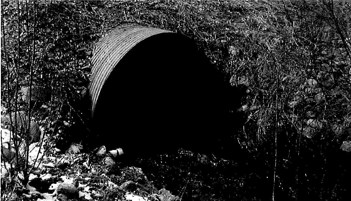
Picture No. 7 is looking at the east downstream end of the 7.5-foot by 11.5-foot elliptical CSP culvert crossing under Noffke Road. Picture is taken looking towards the west.
