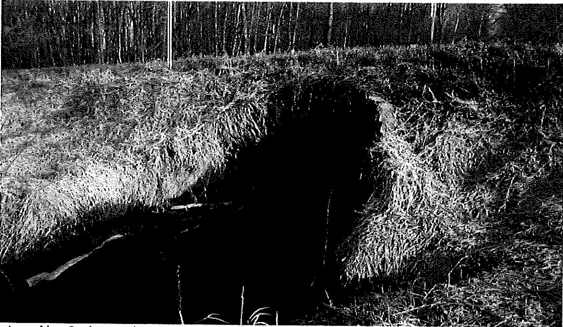
Picture No. 9 shows the southern downstream end of the 8.5-foot by 13-foot arch CSP culvert crossing under 108 th Street. Picture is taken looking northwesterly.
