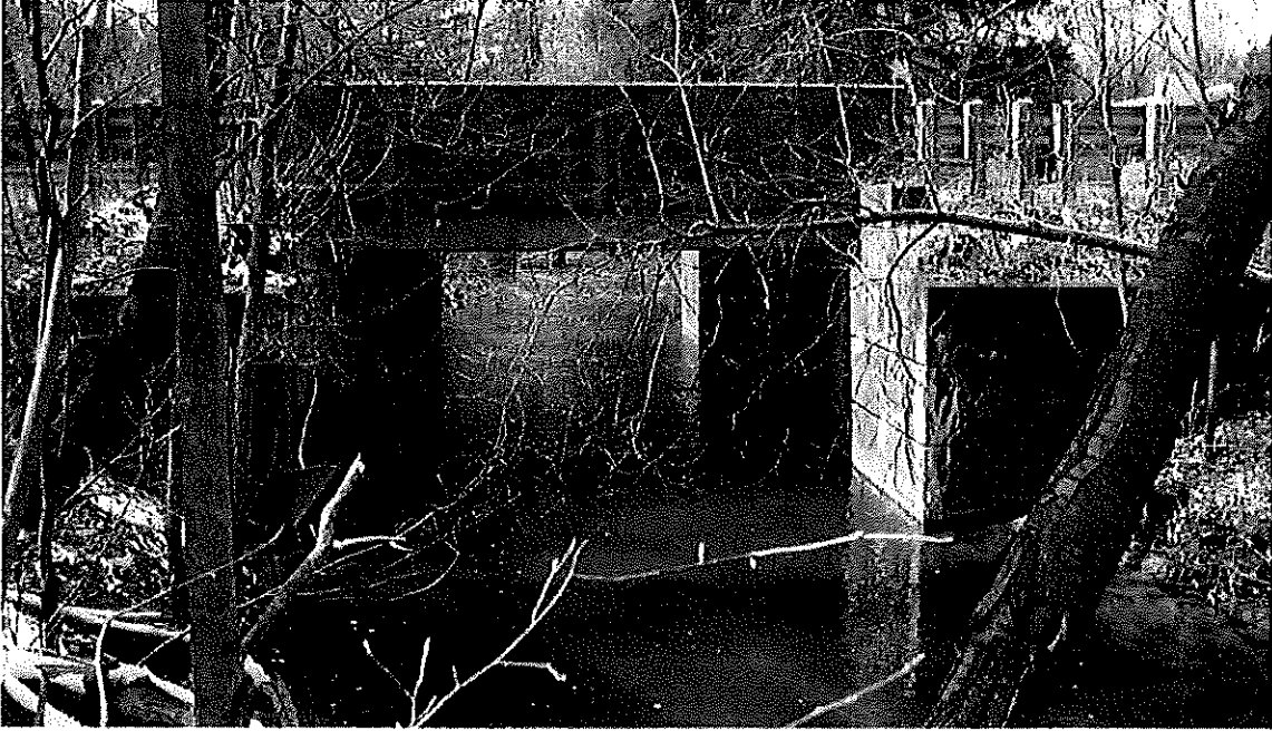
Picture No. 3 shows the eastern downstream end of the 9-foot by 16-foot concrete bridge structure over Cherry Valley Road. Picture is looking towards the west.
