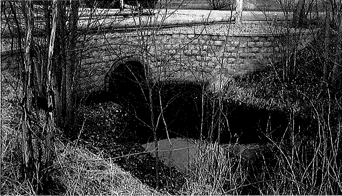
Picture No. 17 shows the eastern downstream end of the 66-inch CSP culvert under Meadow Valley. Picture is taken looking northwest.
