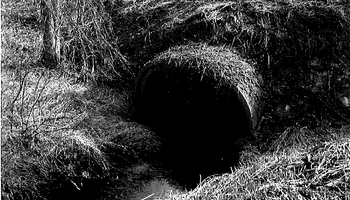
Picture No. 16 shows the upstream western end of the 5-foot by 9-foot elliptical RCP culvert crossing under East Paris Ave.
