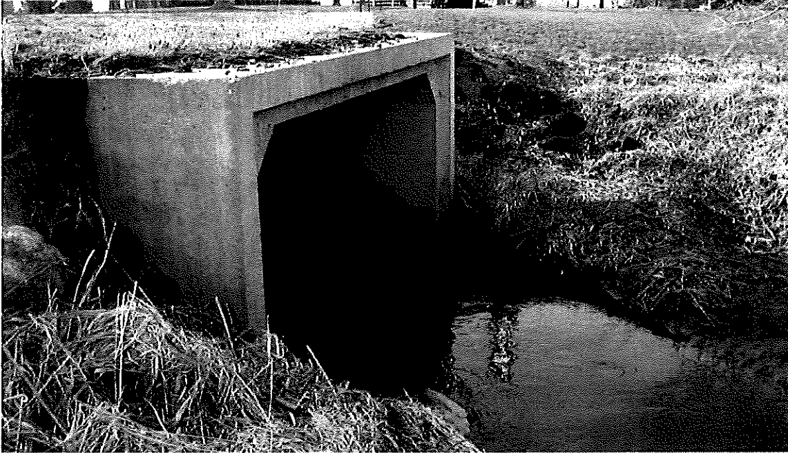
Picture No. 14 shows the western upstream end of the 8-foot by 12-foot concrete box culvert crossing under Patterson Ave.
