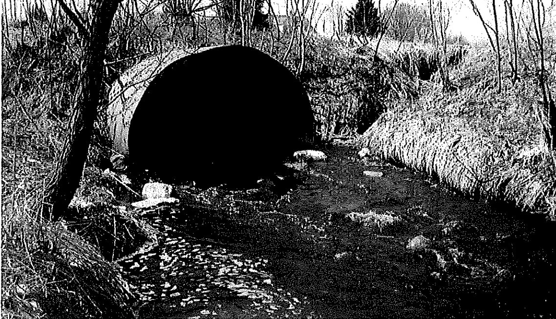
Picture No. 5 is looking west at the downstream end of the 8-foot by 12-foot CSP culvert. Signs of erosion can be seen to the north of the outlet end.
