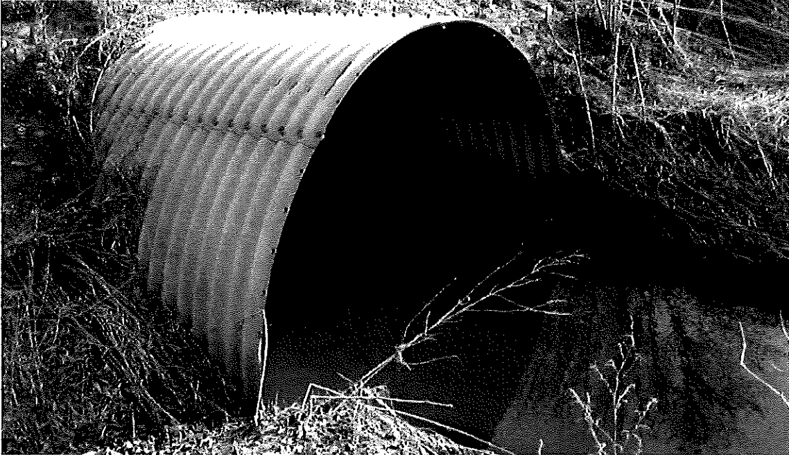
Picture No. 12 shows the southern downstream end of the 9-foot by 12.5-foot arch CSP culvert crossing under 100 th Street.
