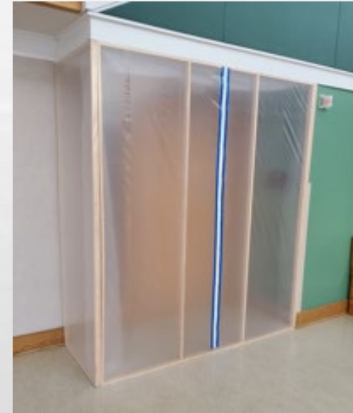
COVID designated— Rehab Center Room with Antechamber at Entry
