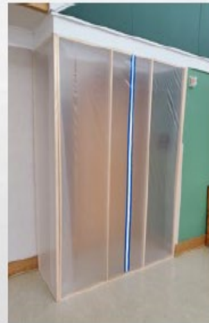
COVID designated— Rehab Center Room with Antechamber at Entry
