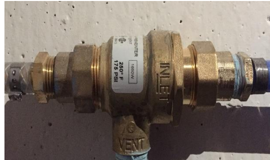
ASSE 1012: Used in place of ASSE 1022 devices except for carbonated beverage machines
