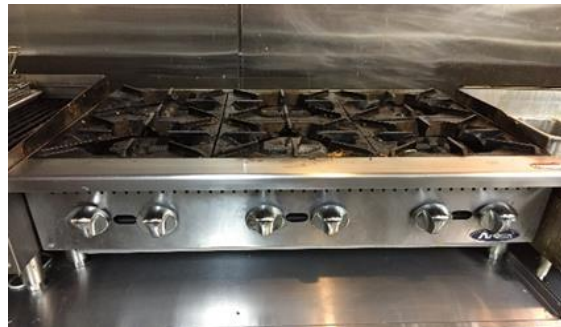
Equipment Elevated 4" Above Counter
