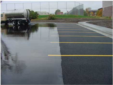
Comparison showing regular asphalt vs permeable asphalt. https://sustainablebuildingsinitiative.org/toolkits/climate-resilience-toolkits/stormwater-mgmt/paving-and-asphalt/toolkit=230
