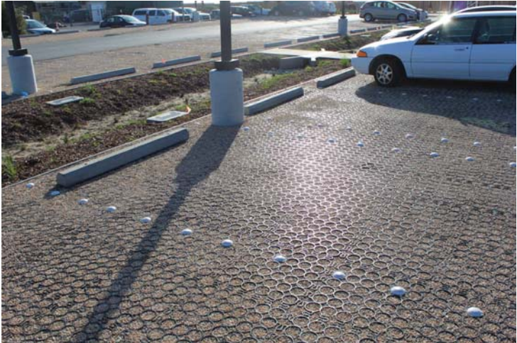
Permeable paving cells are open cells that are filled with gravel or with soil to have grass grown in it. https://www.truegridpaver.com/complete-guide-permeable-paving-systems%E2%82%AC%80/
