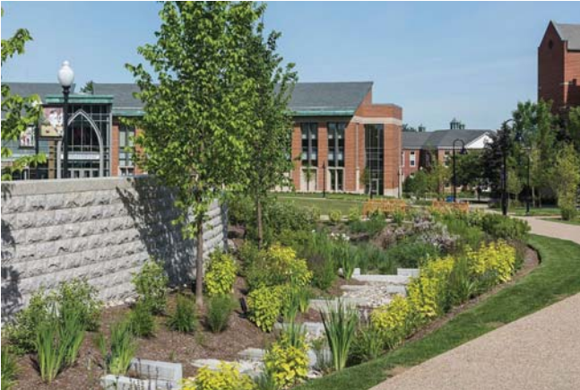
A bioswale at Providence College near the Arthur F. and Patricia Ryan Center for Business Studies. The swale collects water from the road to the left of the image and the surrounding area.
