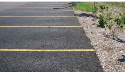
Permeable asphalt along naturalized ditch https://www.freshcoastguardians.com/resources/green-strategies/porous-pavement
