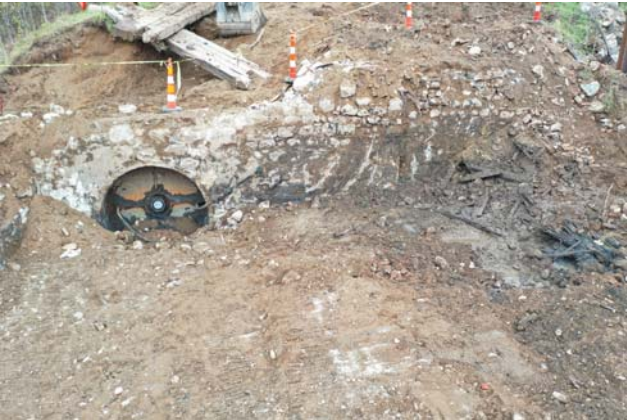
Where the turbine entered the dam structure.
