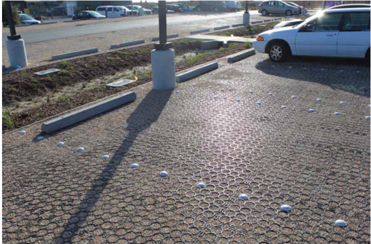
Permeable paving cells are open cells that are filled with gravel or with soil to have grass grown in it. https://www.truegridpaver.com/complete-guide-permeable-paving-systems%EF%BB%BF/
