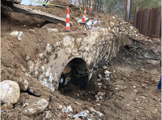
Where the turbine entered the dam structure.
