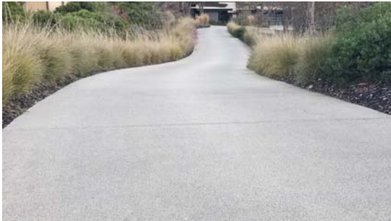
Pervious concrete by Bay Area Pervious Concrete http://www.bayareaperviousconcrete.com/
