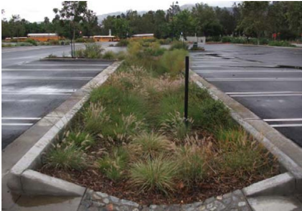
A bioswale in the parking lot at the LA Zoo, both sides of the parking lot drain into it. Image from https://www.canr.msu.edu/news/bioswales_can_improve_water_quality_resources
