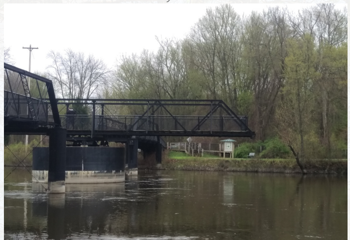
Pictured above: New Richmond Turn Bridge
