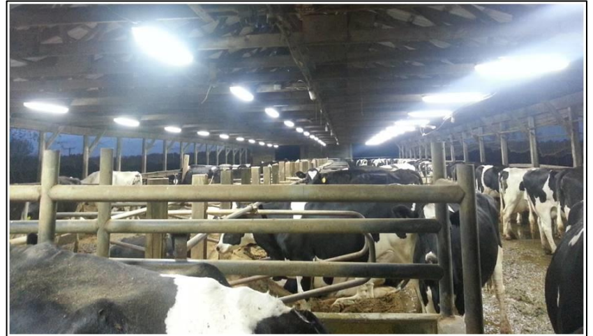
LED lights in barn at Wing Dairy, Barry County, MI
